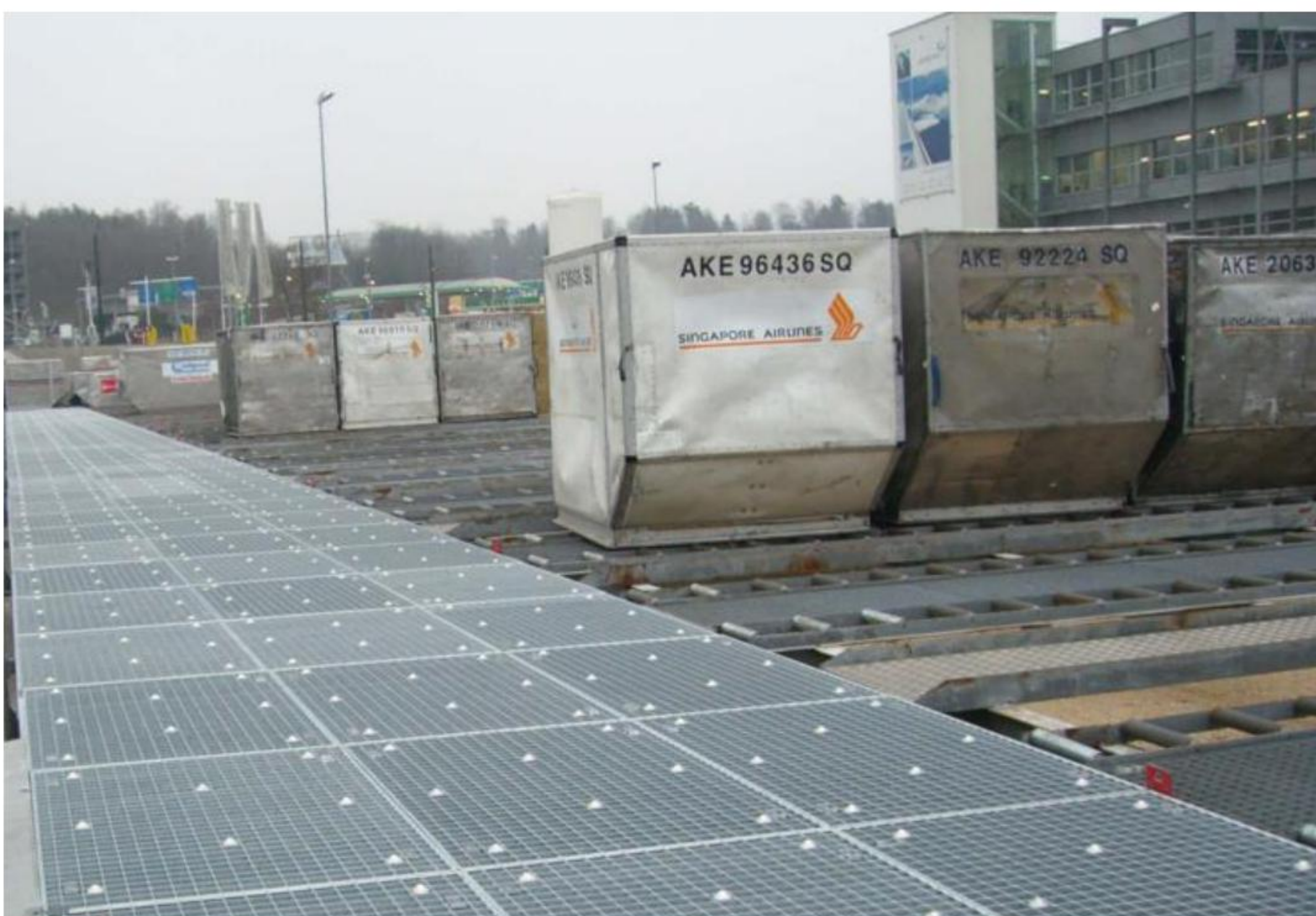
Ball Transfer Units Deck for ULD Zurich Airport
